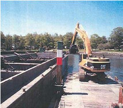
The Mamaroneck Harbor dredging in New York was performed for the New York District Army Corps of Engineers. While not a large project, it posed the challenge of working in a shallow, narrow channel – one that needed to remain open for marine traffic every minute of every day. JCI used the 375 Caterpillar hydraulic excavator dredge. The work needed to be scheduled in tandem with traffic. No problems were encountered excavating 170,000 cubic yards of sediment in 3½ months.
