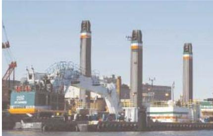
container ports in the world. Part of an aggressive improvement project, this phase increased the depth to 45 feet and generated approximately 1.5 million cubic yards of material. Of that volume, roughly 200,000 cubic yards of pre-characterized contaminated sediments considered unsuitable for ocean disposal were processed and placed at a designated upland disposal site. The remaining
