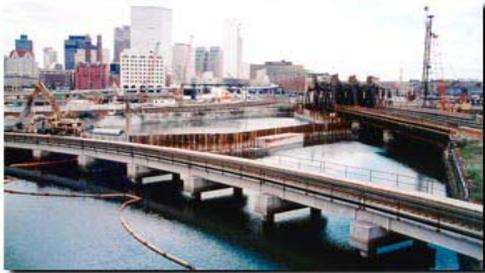
This area of the channel is subject to a 9-foot tidal range and is only 50 feet wide. In Fort Point Channel the contamination was predominantly low-level TPH, with varying degrees of metals but mostly lead and arsenic. These materials were transported by barge to Spectacle Island where they were either processed with cementitious materials or amended with other soils prior to placement
