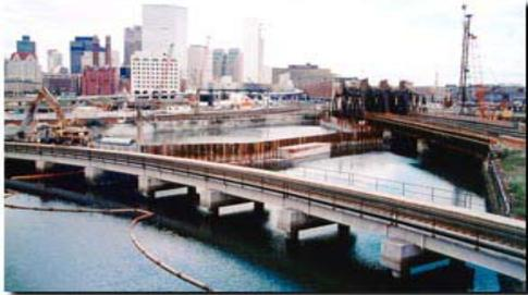
This area of the channel is subject to a 9-foot tidal range and is only 50 feet wide. In Fort Point Channel the contamination was predominantly low-level TPH, with varying degrees of metals but mostly lead and arsenic. These materials were transported by barge to Spectacle Island where they were either processed with cementitious materials or amended with other soils prior to placement
