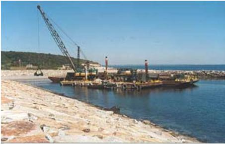
The Pilgrim Nuclear Power Plant Dredging project (40,000 cubic yards) in Plymouth, MA required precision dredging at the plant's cooling water intake structure. The turbidity controls were very stringent, due to concerns with plant turbines. Cashman employed turbidity-removal techniques successfully developed on past projects.
